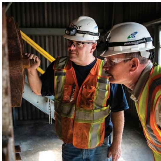
Russell Marshall (left) and Cliff Harmon inspect equipment during the Dale Station demolition project.
