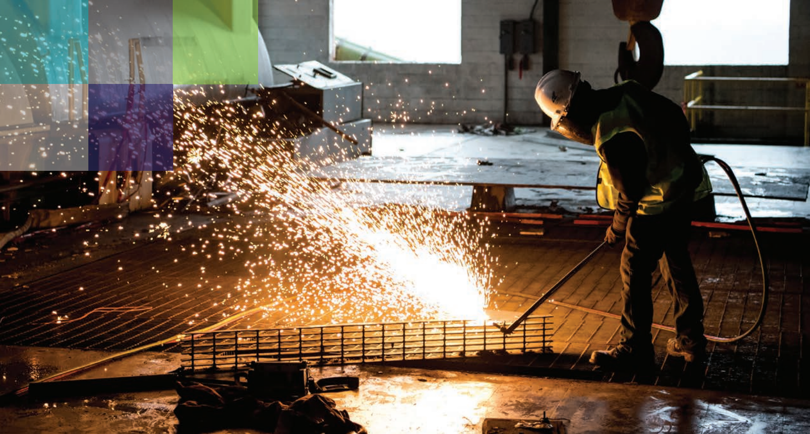
A worker helps in the initial phase of a demolition project to remove the powerhouse and stacks at Dale Station, EKPC's first power plant.
