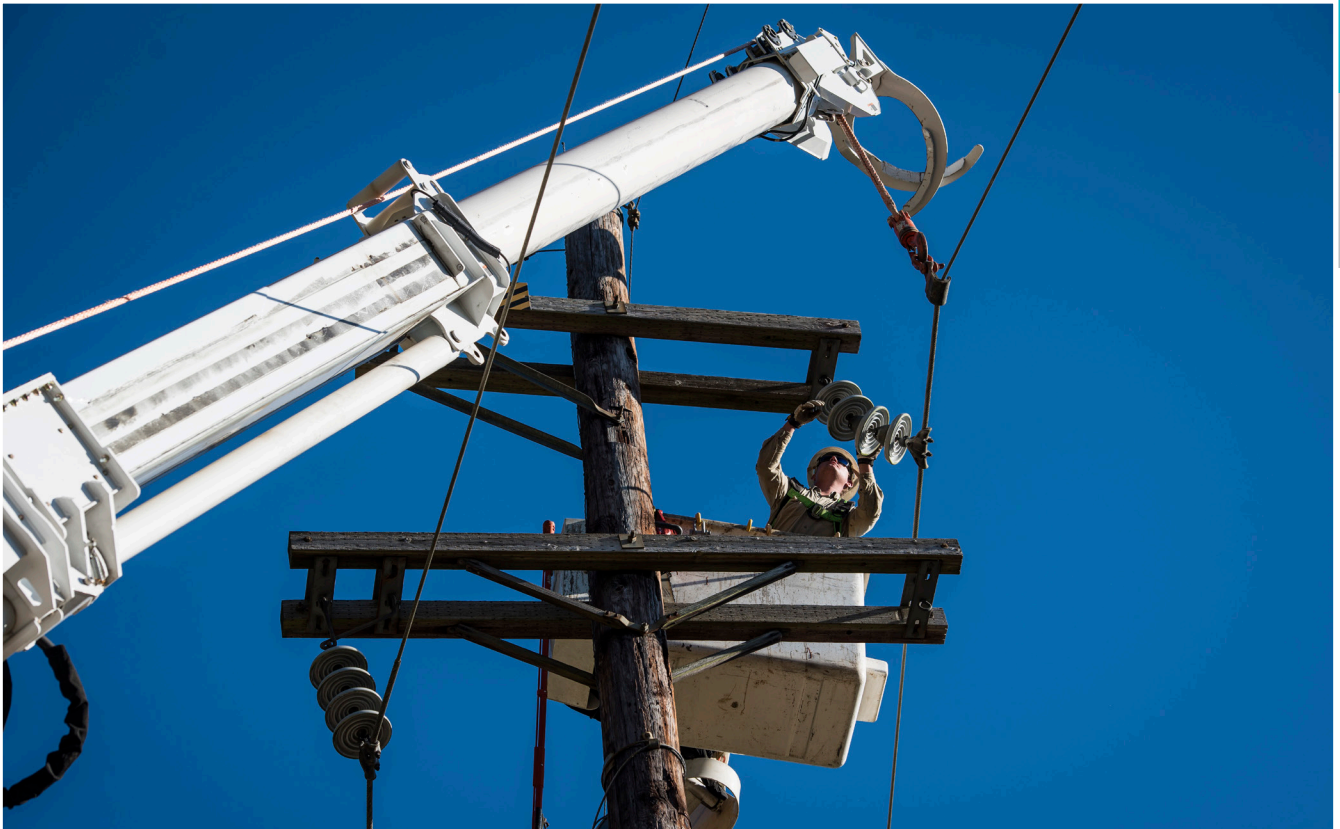
EKPC invested more than $45 million to upgrade the power delivery infrastructure in 2019.
