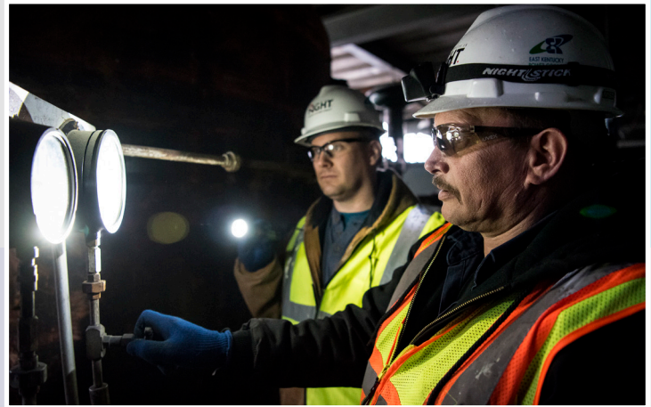
Brent Wasson, left, and Cliff Harmon discuss work being done during the Dale Station demolition.
