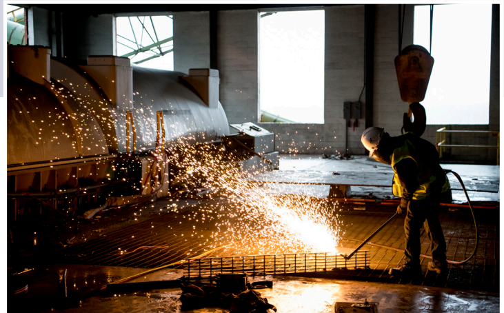
The Dale Station demolition leveled the footprint of EKPC's first power plant.
