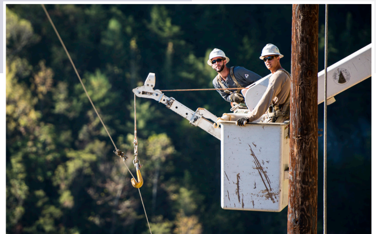
Linemen T.J. Sublett and Blake Polson work on a project in Eastern Kentucky.
