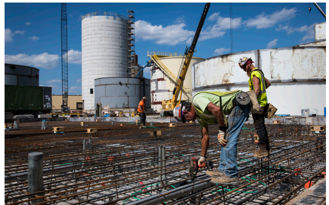
Contractors worked throughout the summer and fall on the project.
