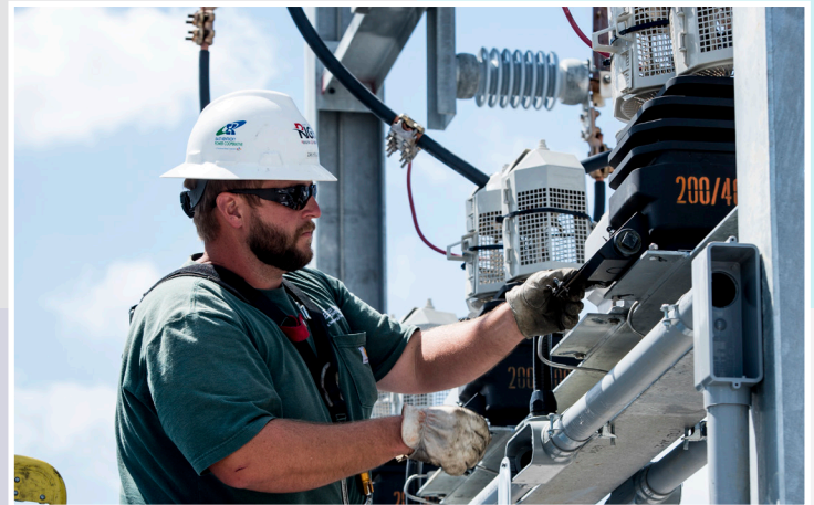
Construction Technician Zach Kelley works on the Hunt Switching Station in rural Clark County.
