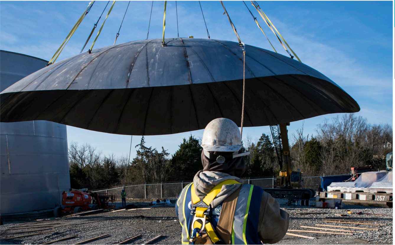
Workers lift the massive top of a new diesel fuel tank at Bluegrass Station.
