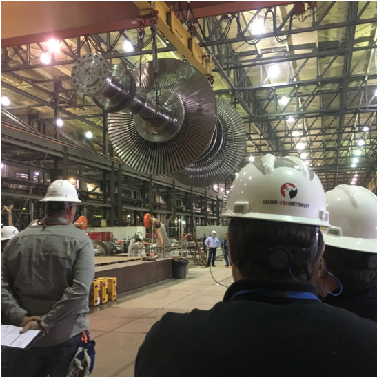
Near the end of the largest outage in EKPC history, workers lift the Unit #4 turbine back into place.
