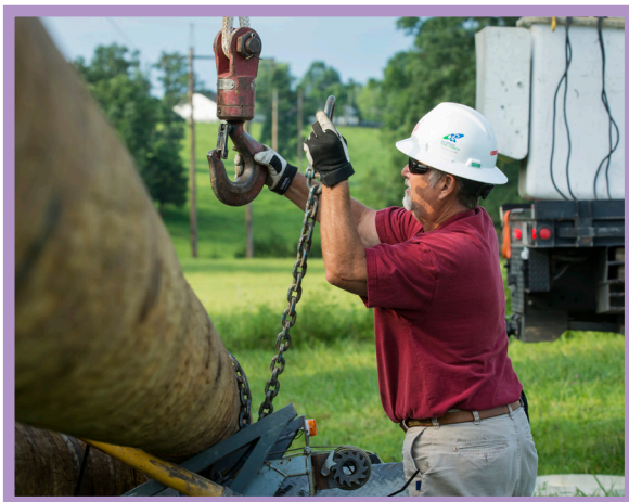
Wayne Prewitt of the Winchester Service Center works to lift a transmission pole.
