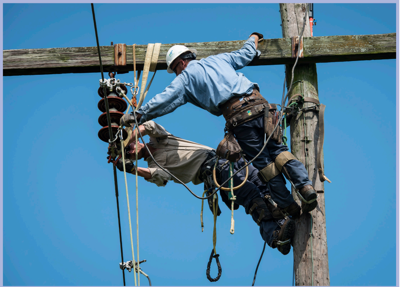
Bardstown Service Center employees work on a transmission line. EKPC invested $22.1 million in 2017 to ensure continued high reliability to owner-members.
