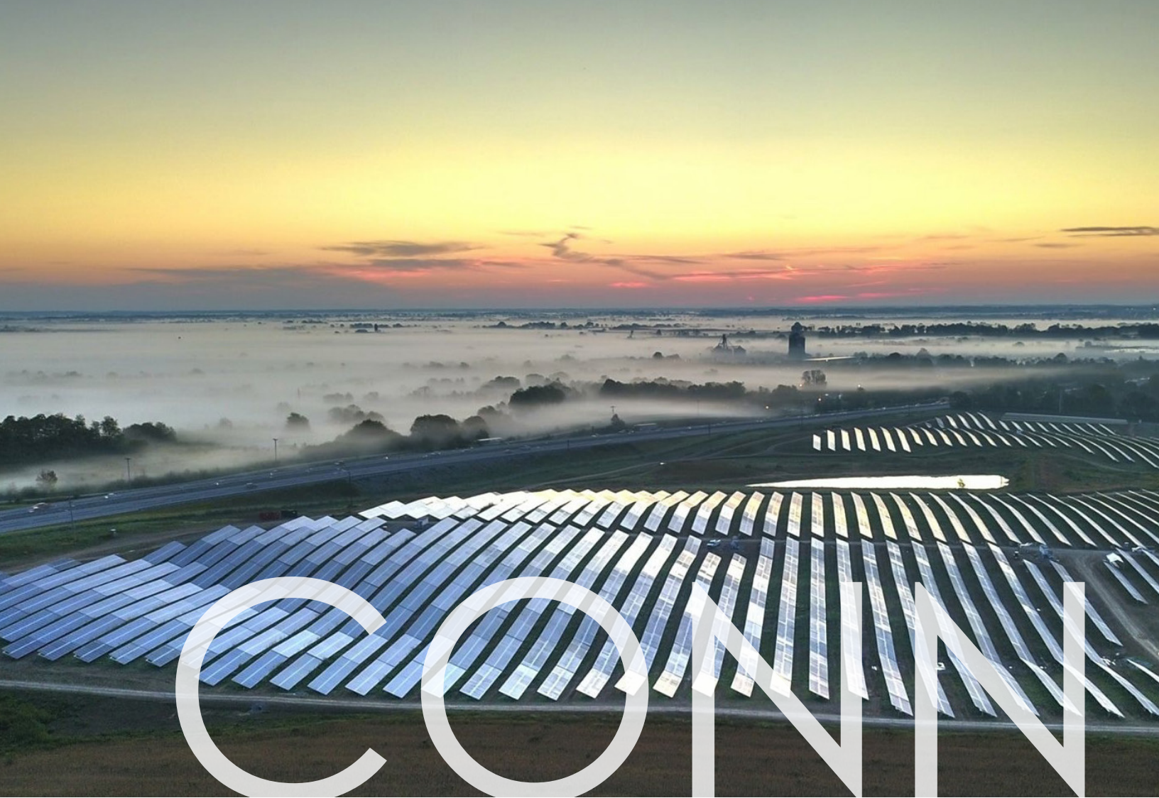
The sun rises on Cooperative Solar Farm One, which was built by EKPC in 2017.
