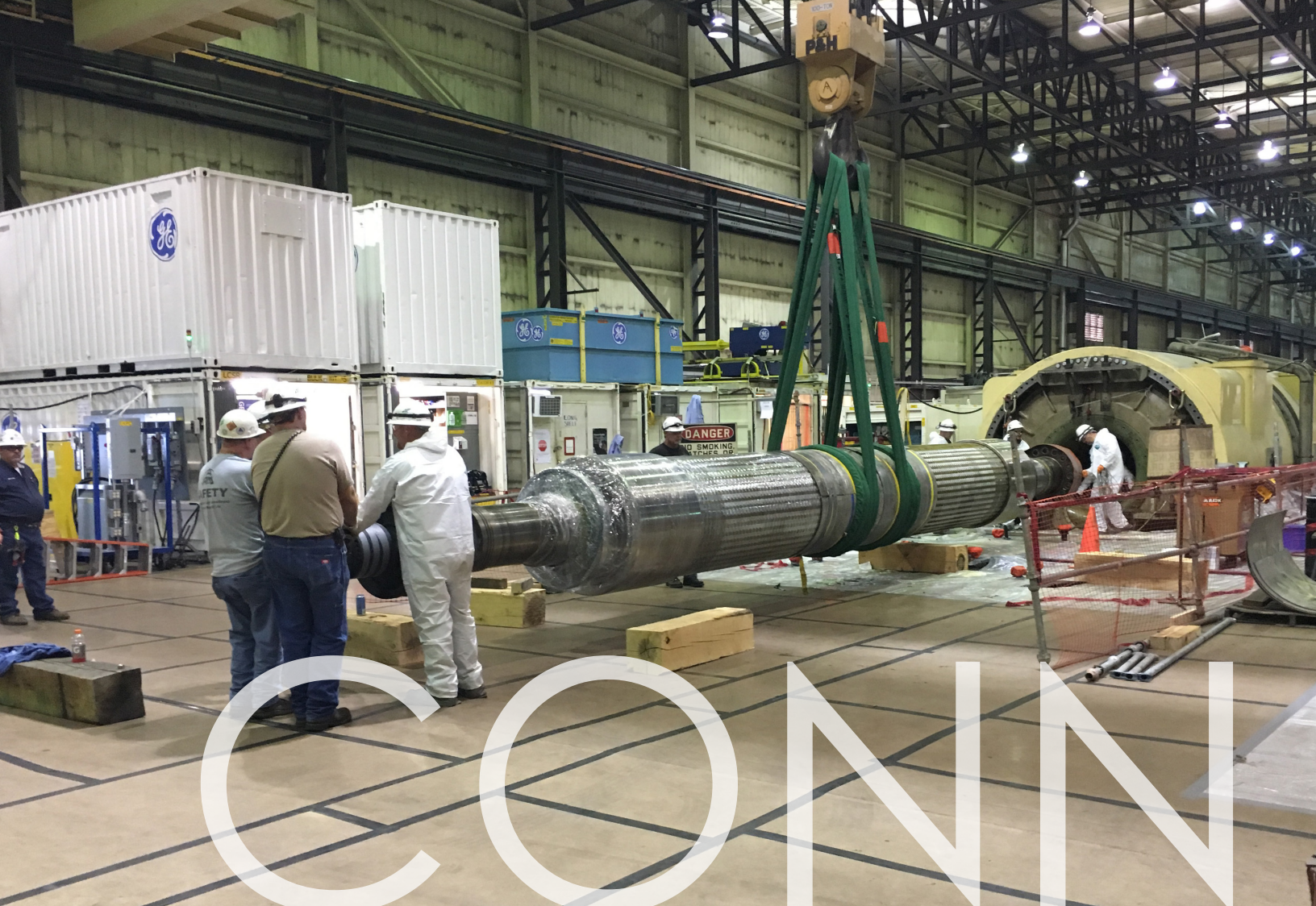
Employees remove the generator field rotor of Spurlock Unit #2 as part of the largest maintenance outage in the history of the cooperative.
