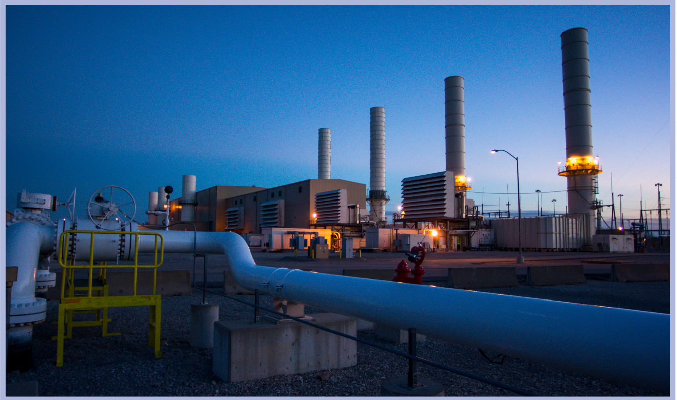
Smith Station in Clark County has nine natural gas fueled units that help EKPC to meet peak system demand.
