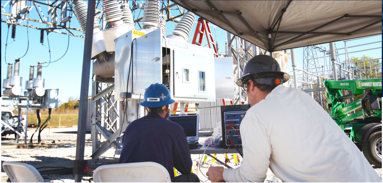
A new vacuum breaker is installed in Barren County. The vacuum breaker technology is being piloted to replace sulphur hexafluoride gas breakers, which is a powerful greenhouse gas.
