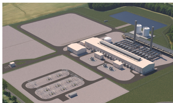
This is a rendering of the 214-megawatt RICE facility which will be built in Liberty, KY in 2026 with operations by 2028.
