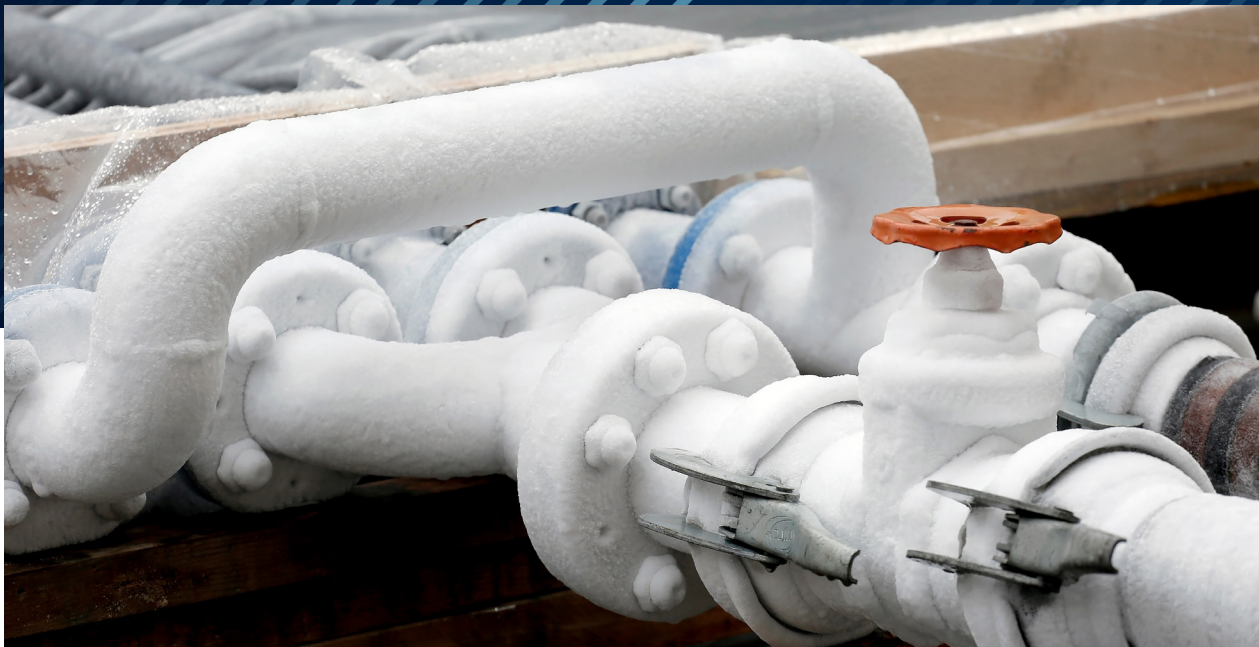
Frozen pipelines during Winter Storm Elliott caused difficulties starting the gas units.
