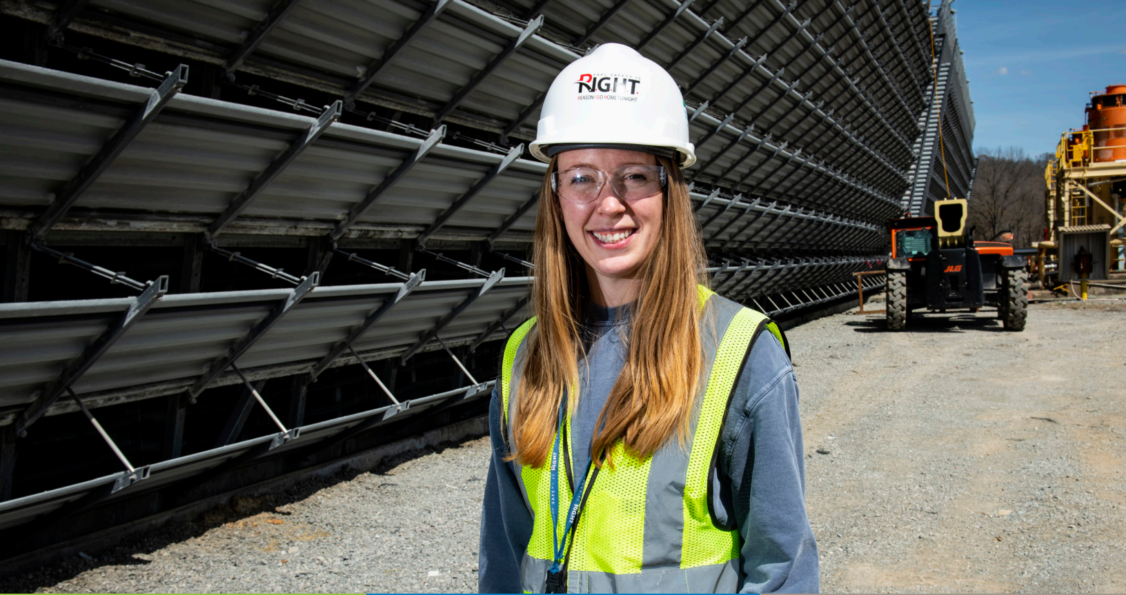
The water cooling tower construction at Spurlock Station.
