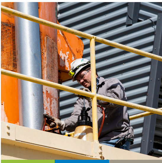
Construction of the wastewater treatment plant at Spurlock Station.
