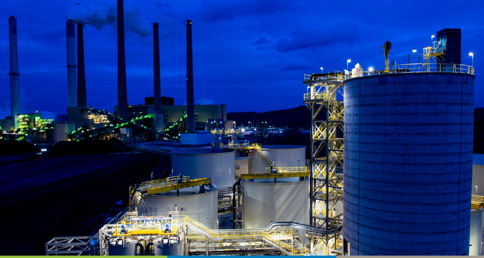
Spurlock Station completed a new wastewater treatment facility in 2021.
